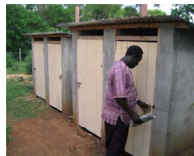
New latrines at the Obambo clinic
