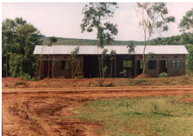
The new clinic in Obambo under construction
